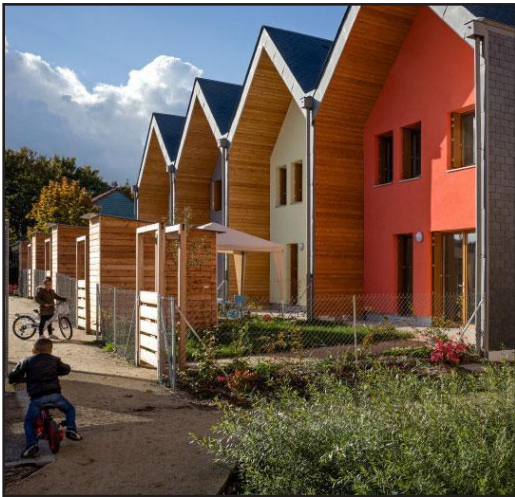
Ecoquartier des Noés / APM Architecture Val-de-reuil, France
